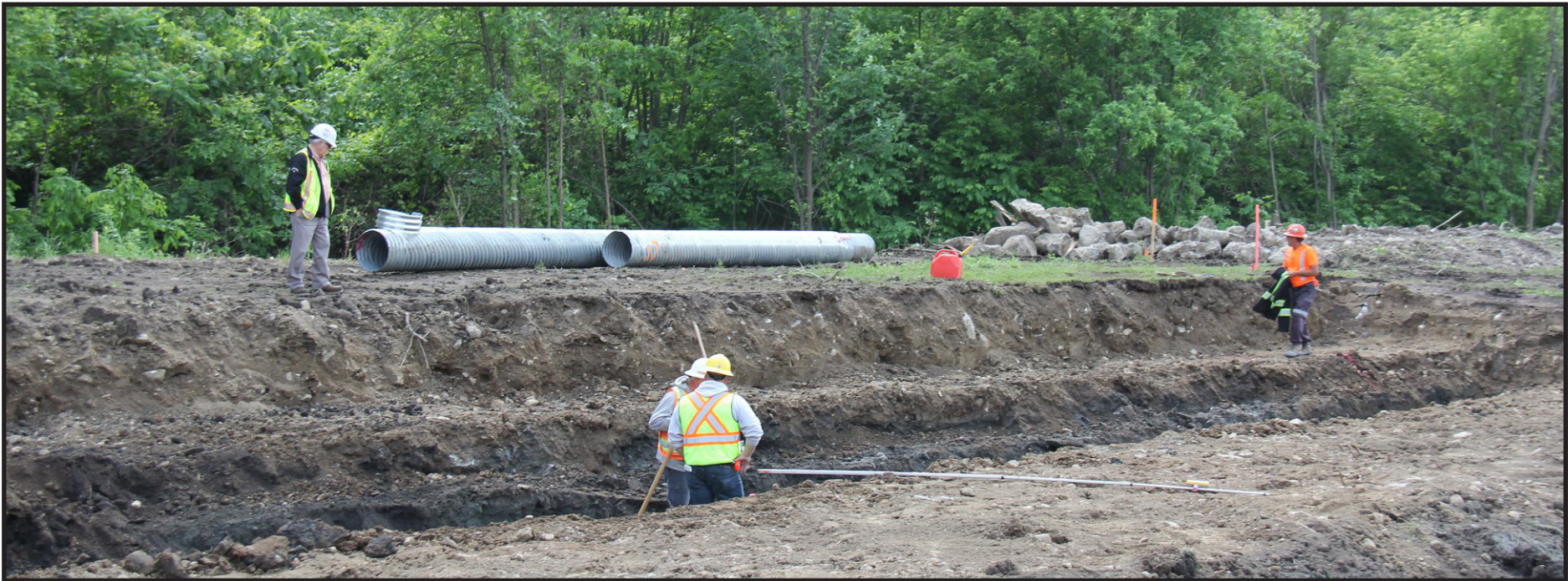
The culvert pipes that are being installed are used to provide drainage in order to prevent flooding.
