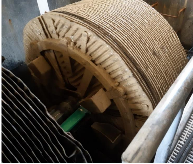
Heavy alum build up on bank one in 2018 prior to media failure
