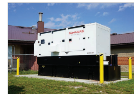
Generator installation at Iakhihsotha Lodge.
