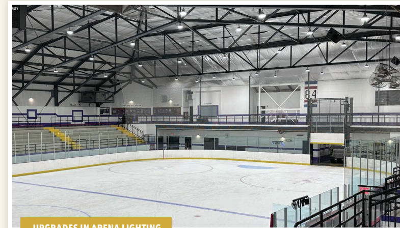
UPGRADES IN ARENA LIGHTING
