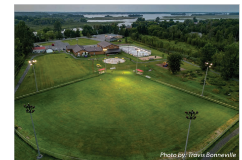
Snye Recreation ballfield lighting upgrades. Photo by: Travis Bonneville
