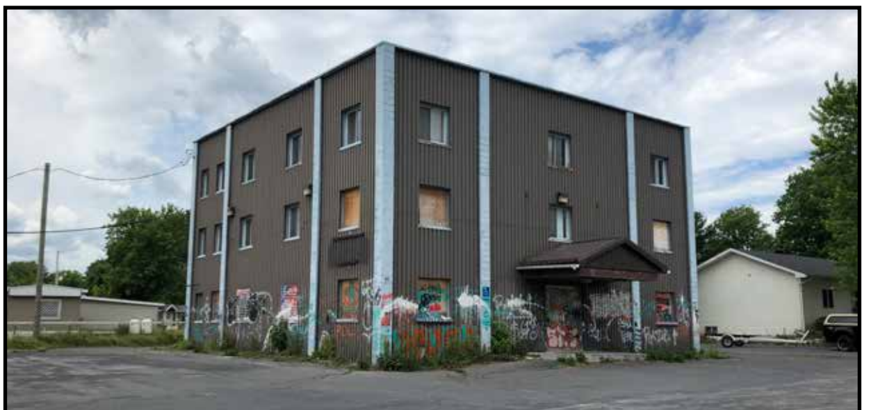
The former Administration 2 building will be soon be demolished.
